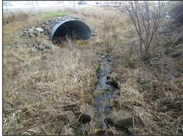
Site 7: Facing east (downstream) at upstream end of 407 ETR culvert downs rocky ramp (Spring 2019).
