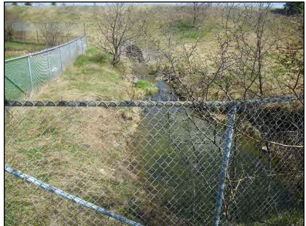
Site 4: Facing northeast (downstream) from the pipe outlet at Guelph Line (Spring 2019).
