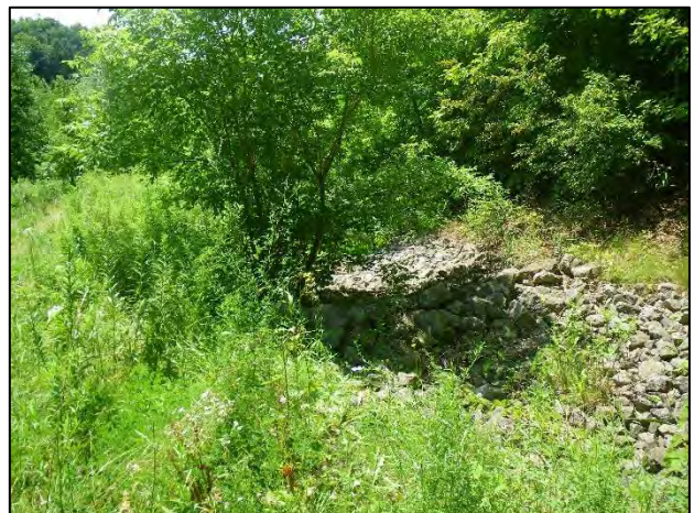
Site 30: Facing south (downstream) at rip rap slope further downhill (Summer 2019).
