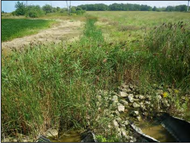
Site 24: Facing east (downstream) from 407 ETR culverts (Summer 2018).
