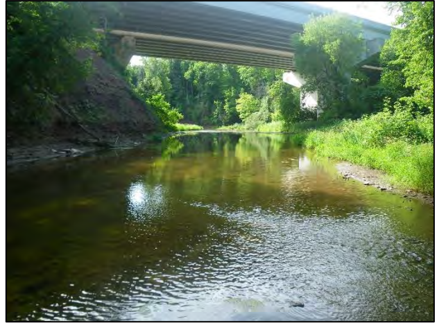
Site 15: Facing south (downstream) at the 407 ETR bridges (Summer 2019).
