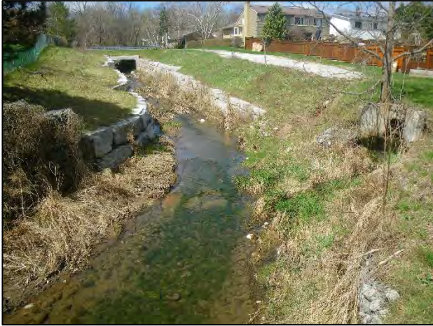
Site 2: Facing west (upstream) from upstream of 407 ETR culvert (Spring 2019).
