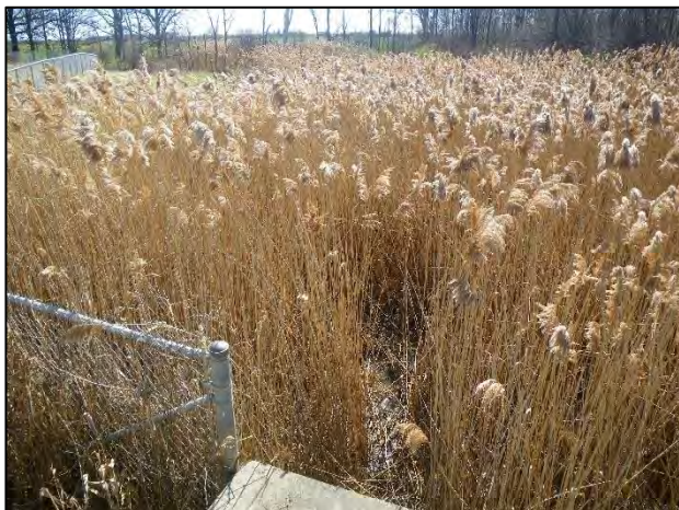
Site 39: Facing east (downstream) from the 407 ETR culvert (Spring 2019).
