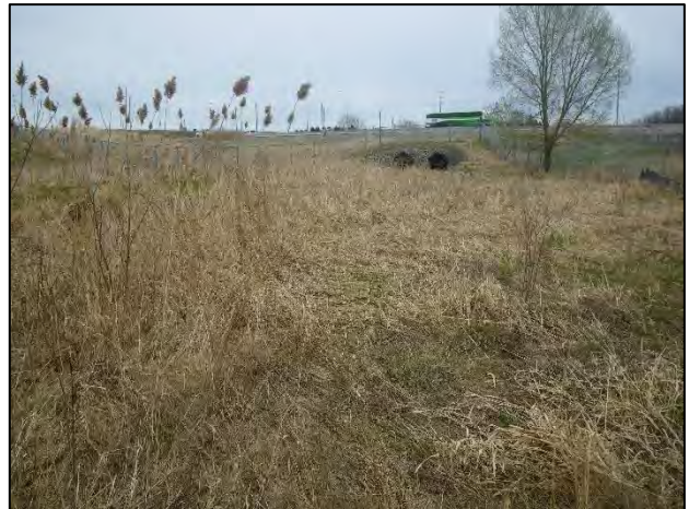
Site 16: Facing east (downstream) at the 407 ETR culverts (Spring 2019).
