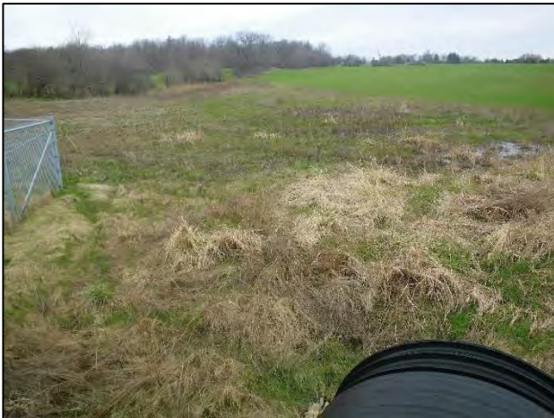
Site 14: Facing northwest (upstream) from 407 ETR culvert (Spring 2019).
