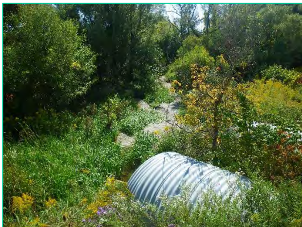
Site 52-54: Facing southwest (downstream) from the 407 ETR culverts (Summer 2019).
