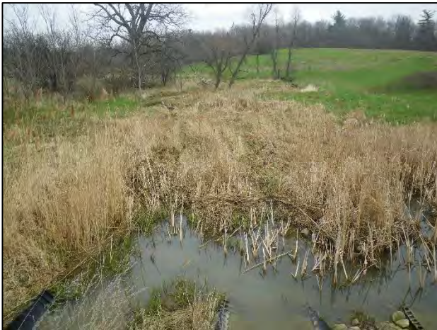
Site 22: Facing east (downstream) from the 407 ETR culverts (Spring 2019).
