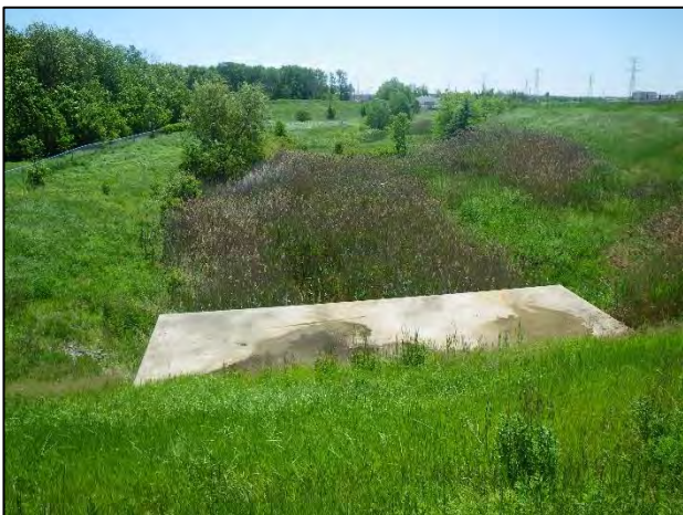
Site 44: Facing southwest (downstream) from the Derry Road culvert (Spring 2019).
