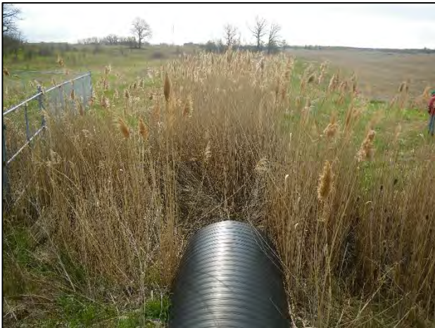
Site 19: Facing southeast (downstream) from the 407 ETR culvert (Spring 2019).
