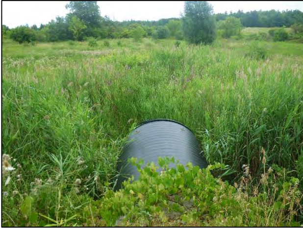
Site 28: Facing east (downstream) from 407 ETR culvert (Summer 2019).
