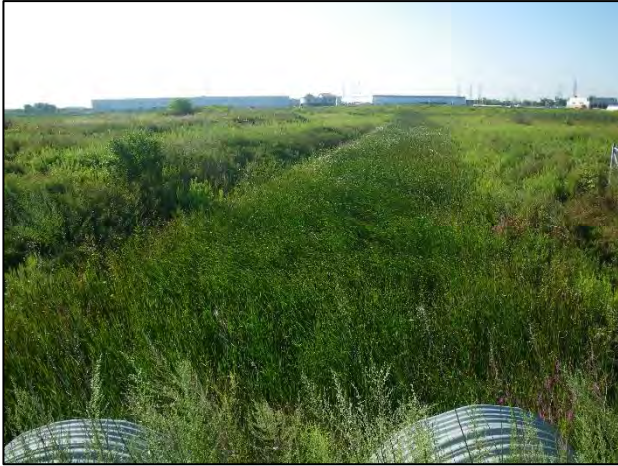
Site 47: Facing south (downstream) from the Hwy 401 EBL to 407 ETR EBL ramp culverts (Summer 2018).
