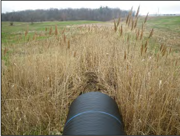
Site 21: Facing southeast (downstream) from the 407 ETR culvert (Spring 2019).
